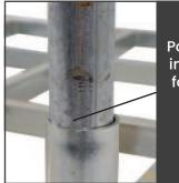
Poles slide into base for quick setup
