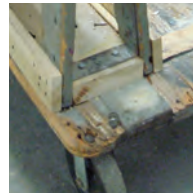
Wood—splinters and rot
